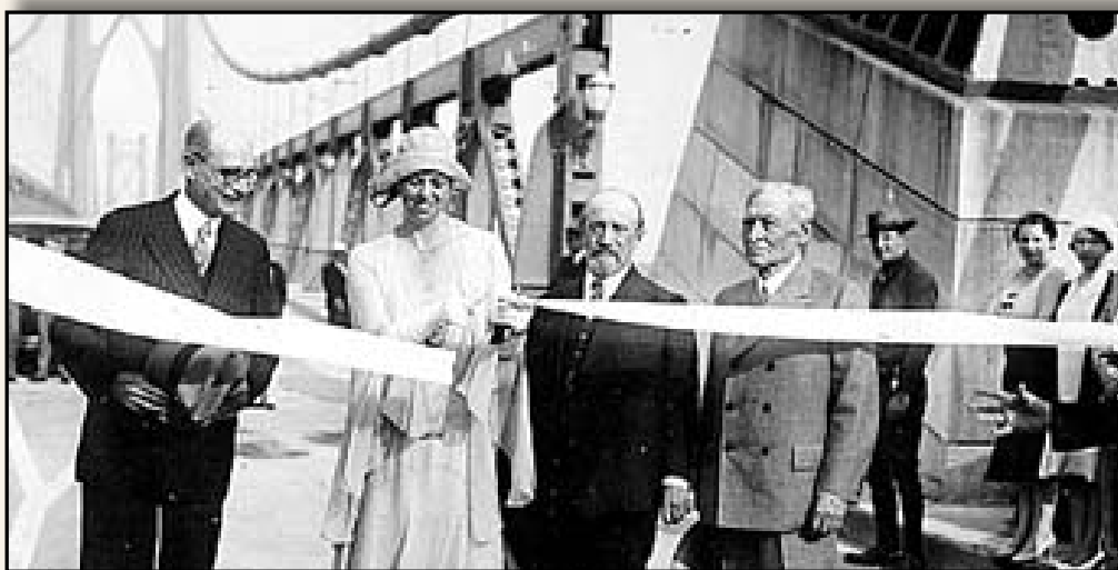
Opening of the (Roosevelt) Mid-Hudson Bridge, 1930
